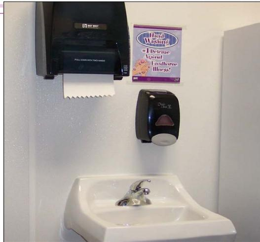
A handwash sink may be any type of freestanding sink with soap and paper towels available. The Ohio Uniform Food Safety Code does not permit handwashing in the three-compartment sink.
